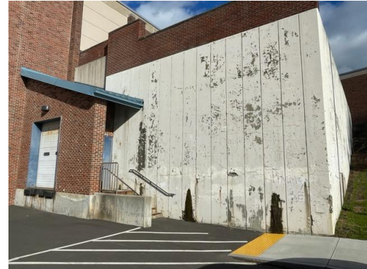
Repair damaged concrete wall at Central Receiving
