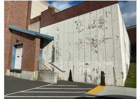
Repair damaged concrete wall at Central Receiving
