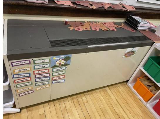
Replace unit ventilators in classrooms
