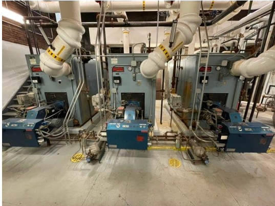
Replace existing boilers
