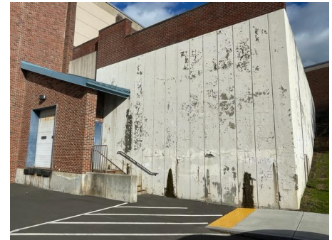
Repair damaged concrete wall at Central Receiving
