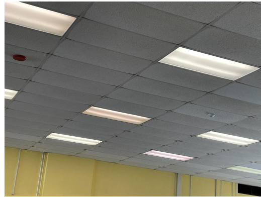
Replace old lights with LED lights
