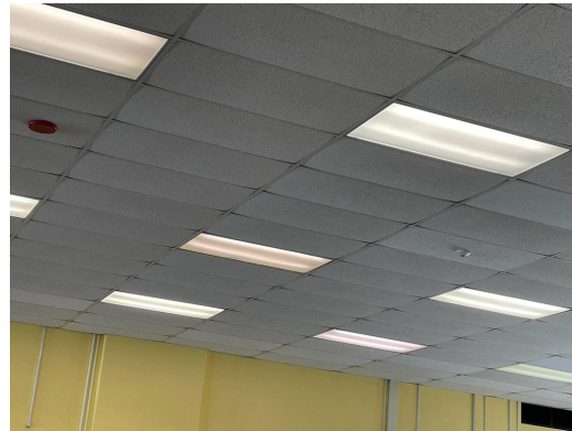
Replace old lights with LED lights
