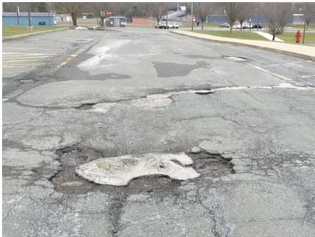
Paving of parking lots and driveways
