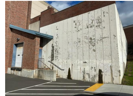
Repair damaged concrete wall at Central Receiving
