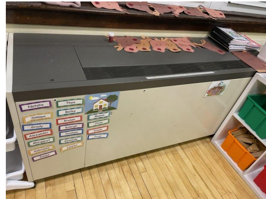
Replace unit ventilators in classrooms
