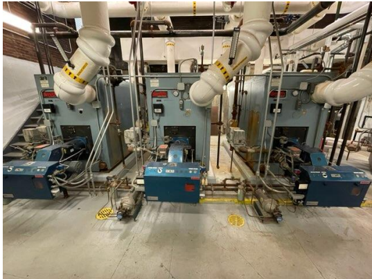
Replace existing boilers
